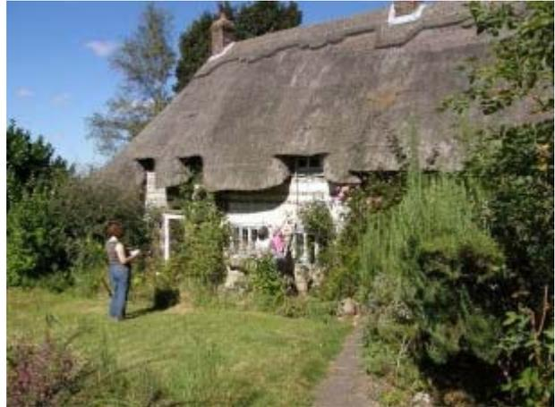
The materials and methods of construction of both the roof and walls should be taken into account. A tiled roof with a pitch of 47 degrees or greater was probably originally thatched whilst the bond used in the brick work can suggest a building's age and the social pretensions of the owner, some bonds requiring far more bricks than others and entailing much greater expense.
